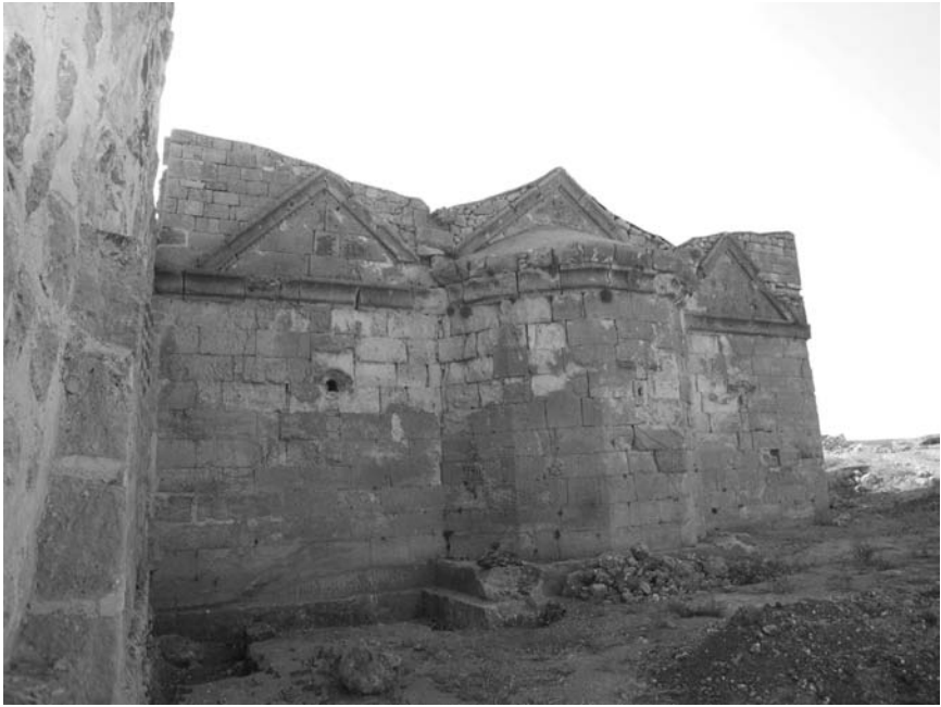
Fig. 3.3.12 Monastery of Mor Ya'qub at Şālah, five-sided apse of the main church
